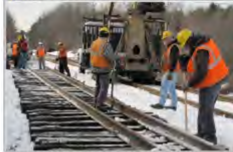
Figure 4-G. Construction of the Downeaster Extension
