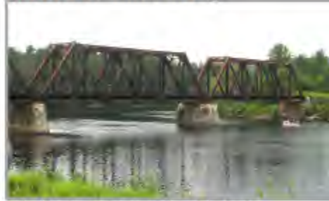
Figure A-1. The Connecticut River Bridge
